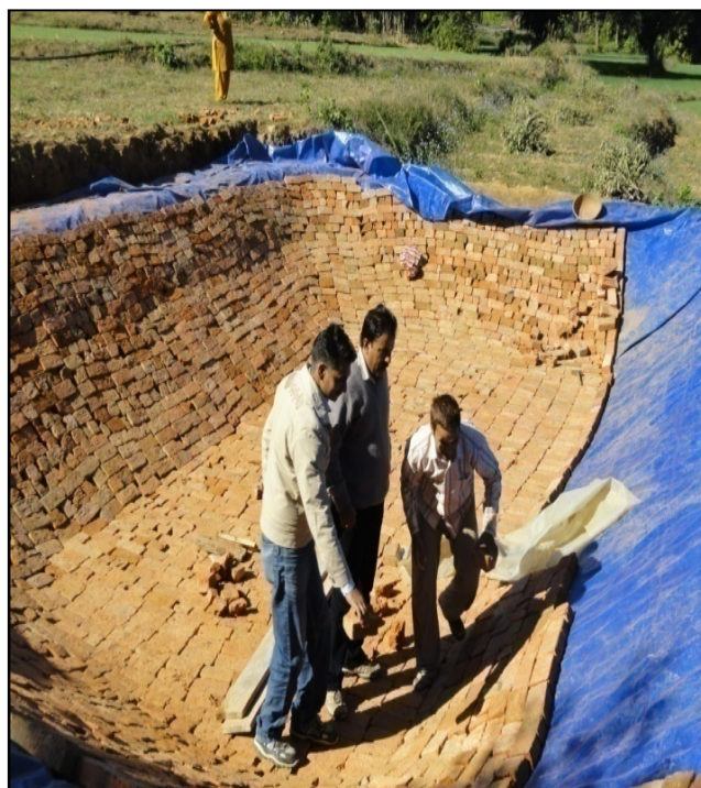
Figure 1: Construction of Silpauline polylined tank.
